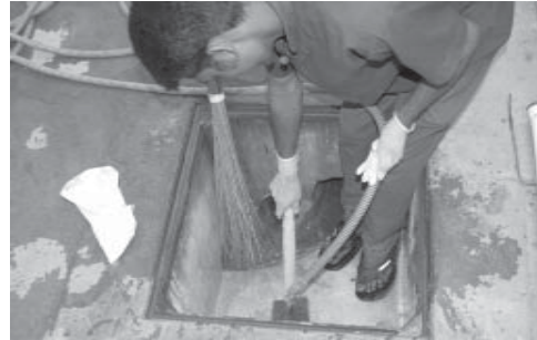
Fig. 13.1 - Cleaning the septic tank connected to a public drain
