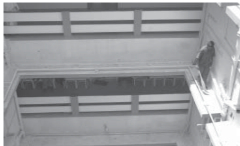
Fig. 6.5 - Cleaning the sunshade
